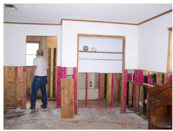
Removing drywall and insulation from a flooded home after Hurricane Ike
